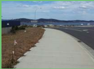
The upgrade of Rokeby Rd, Tasmania included shared paths on the Tollard Drive extension.
