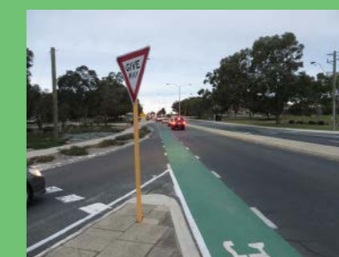
Bicycle lanes were marked along 236m of Winterfold Rd to address issues identified in the City of Fremantle Local Bicycle Plan. The lanes were constructed to provide a dedicated space for cycling and to allow green paint to be used to highlight conflict areas at intersections.
