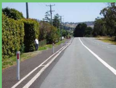
A shared path was constructed along the shoulder of John Lees Drive, Tasmania to improve walking and cycling safety.
