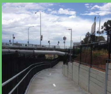
Keswick underpass before (above) and after (below) showing the transformation that was achieved by a $2 million investment in the Marino Rocks Greenway. The underpass forms an important link connecting existing paths on either side of this busy intersection and improves the attractiveness and directness of the Marino Rocks Greenway. The underpass also improves access to the Adelaide Showground station on the Belair, Seaford and Tonsley rail lines. The underpass completed the Adelaide Showground Station project, jointly funded by the Australian and South Australian Governments as part of the Goodwood Junction upgrade.
