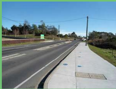
A shared path and refuge crossing was built along Stony Rise Road, Tasmania linking a large residential area with the Devonport Homemaker Centre.
